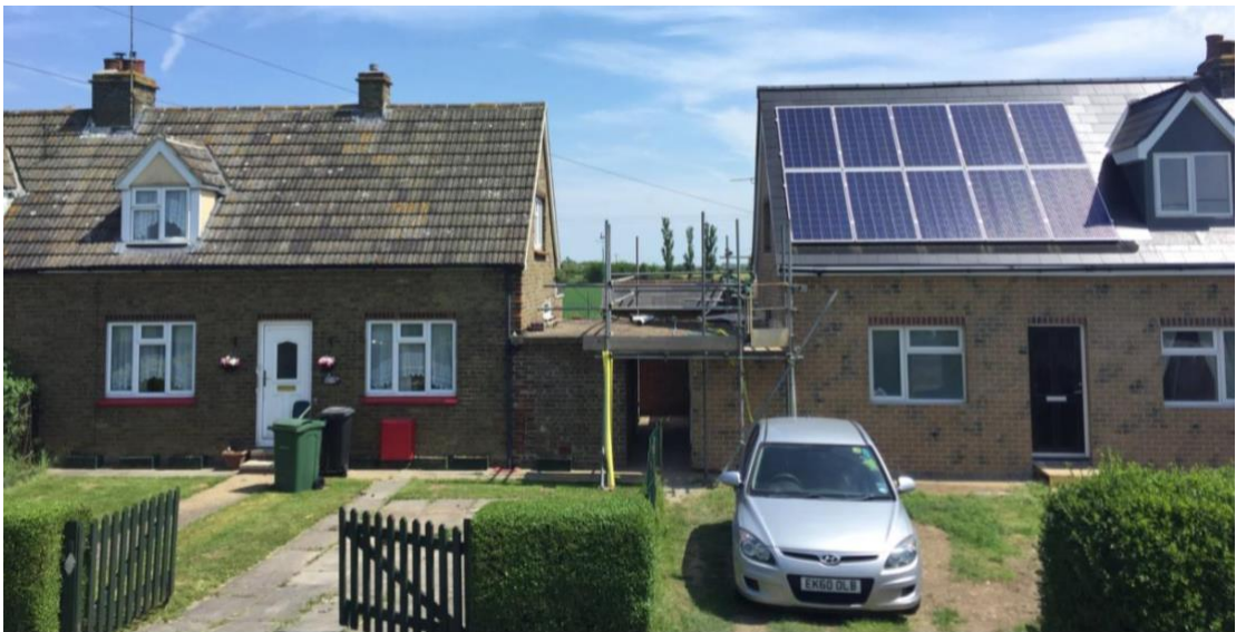
Energiesprong project in Maldon, Essex on right (similar house without on left)
